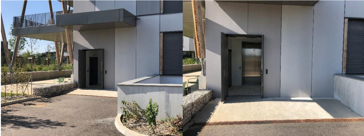
Figure 7-9 – Entrance for bulky material delivery at RTE international in Lyon.
