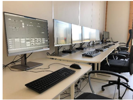
(d) Operator workstation in the operator room
